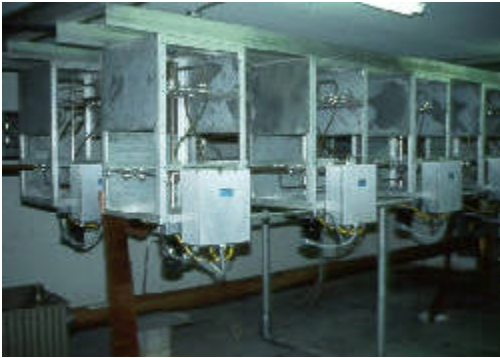
The matrix switch room at a high power short-wave broadcast station.
