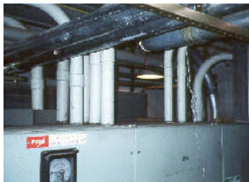
Top of a an electrical switch panel with cables in conduit exiting top of cabinet.
