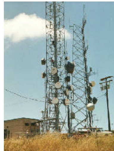
A common communications tower site with microwave, cellular, paging and conventional two-way radio antennas.
